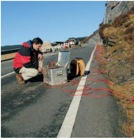
resistivity cable deployment in road verge
